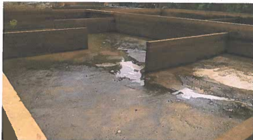
Badli Industrial Area CETP
