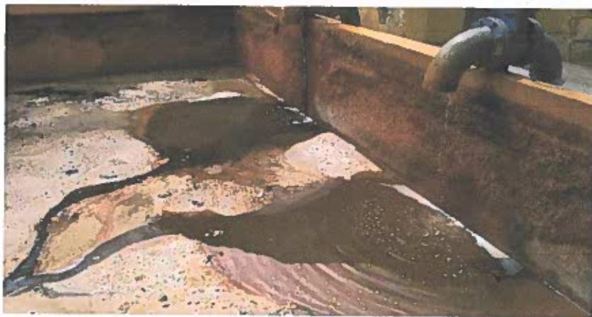
Badli Industrial Area CETP
