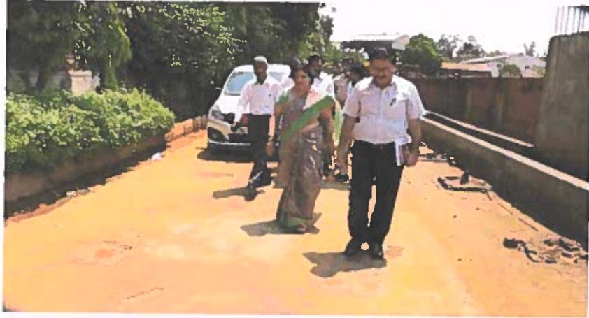
Wazirpur Industrial Area CETP Plant
