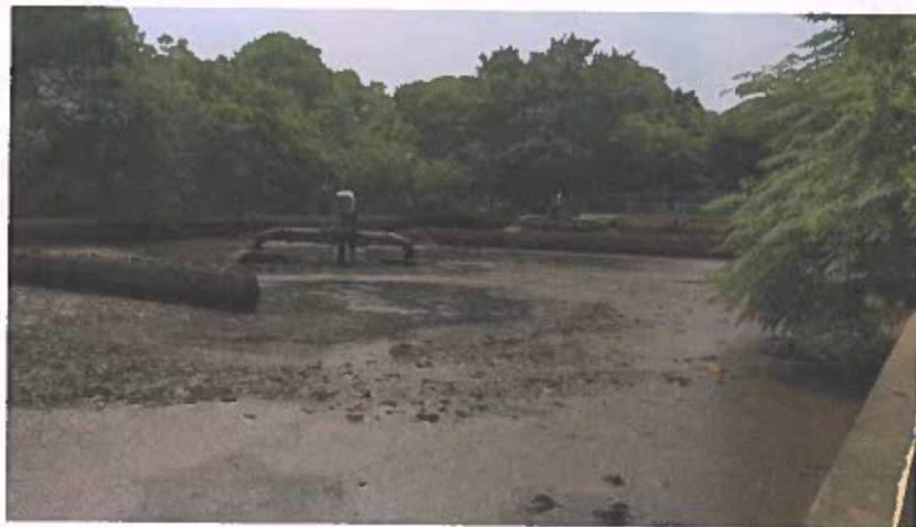
Badli Industrial Area CETP
