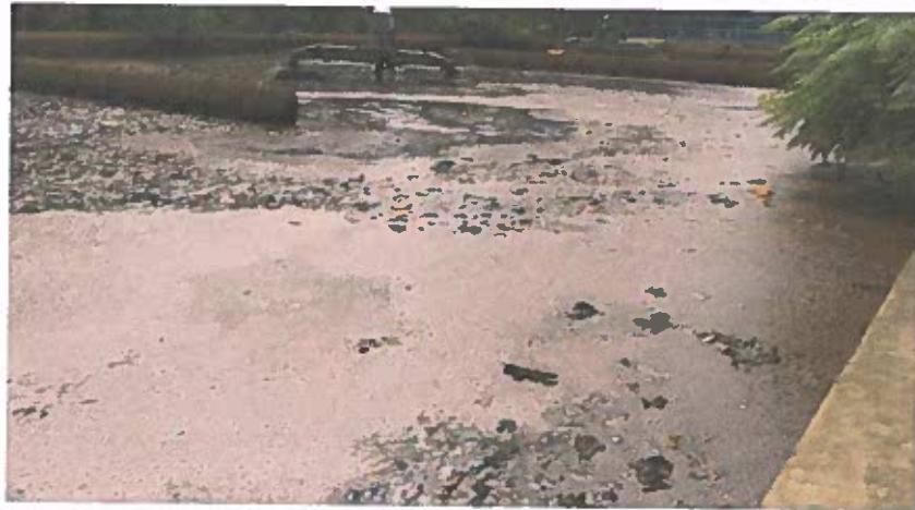
Badli Industrial Area CETP
