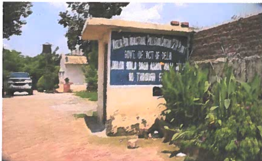
Wazirpur Industrial Area CETP Plant
