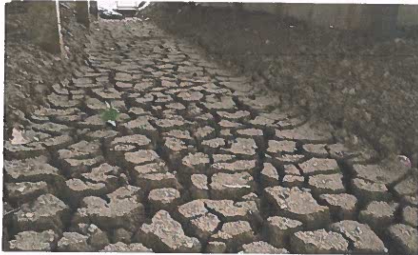
Badli Industrial Area CETP
